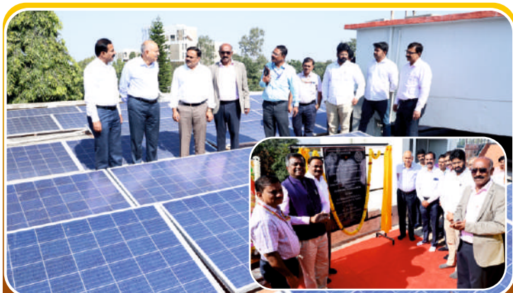
Inauguration of Solar Power Plant on 7 th January, 2025 at CoA, GKVK building by Shri P. Ravi Kumar, IAS (Rtd.), Chairman, KERK, GoK
